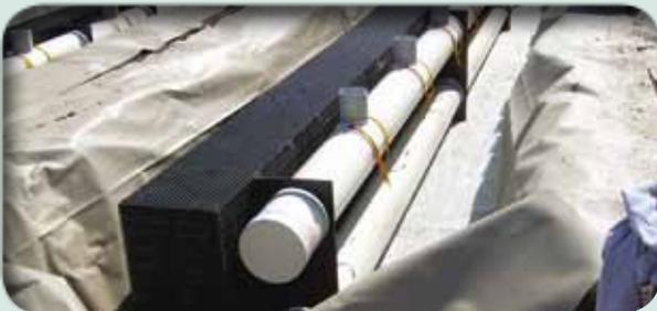
**Step 2:** Clip together the load-bearing plastics crates (recycled car bumpers) which are said to be 98 per cent void. Install the ductwork, locating and supporting them in frames.
