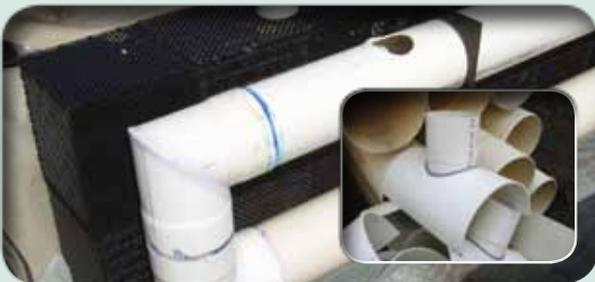
**Step 3:** Cut holes for supply spigots. Inset: The spigots themselves are heat-welded onto collars and sealed into position. Pressure test the ductwork to ensure integrity before filling the water tanks.
