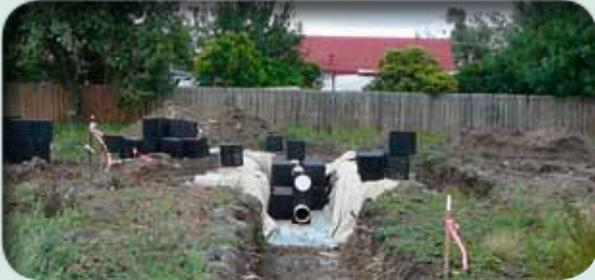
**Step 1:** Dig a trench. Line it with a liner commonly used in Australia to create underground water tanks. The former school on the site used diesel generators, and construction work was delayed while the site was excavated by 2m to remove contaminated soil.
