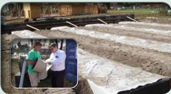
**Step 4:** Wrap up the tanks and seal them once the ductwork sections have been pressure tested. Top-hat sections seal the spigots above and below the water line to the tank liner. These have yet to be welded to the liner over the ventilation spigots, which can just be seen straining against the now-sealed water tanks. Inset: Architect Neville Cowland checks the seal of the top-hat sections with the contractor.
