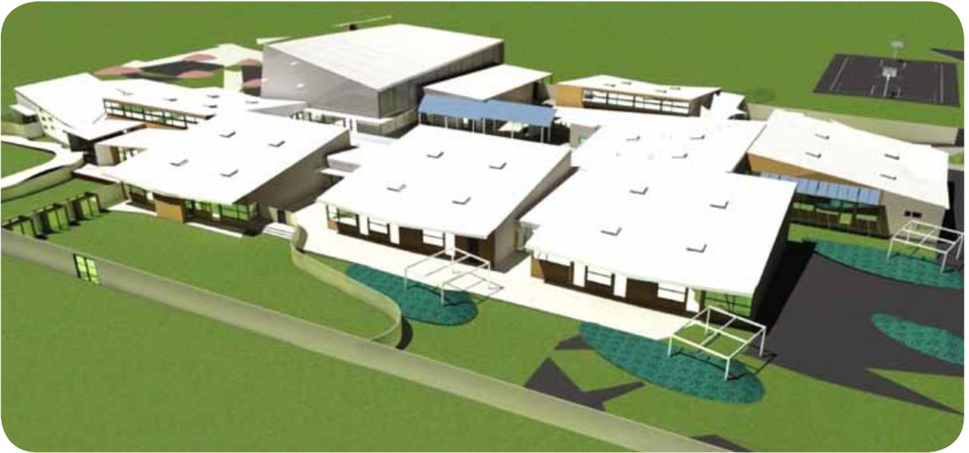
The school's plan is formed by combining modules whose cross-sectional shape induces airflow. The long walls of the gymnasium will be formed by a dual skin of translucent corrugated fibreglass sheet. This aims to give even natural lighting during the day and allow heat harvesting or rejection by flap controls.
