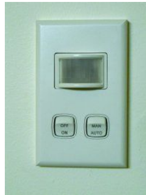
Lighting can be switched between automatic and manual control using very intuitive and well-labelled switches
