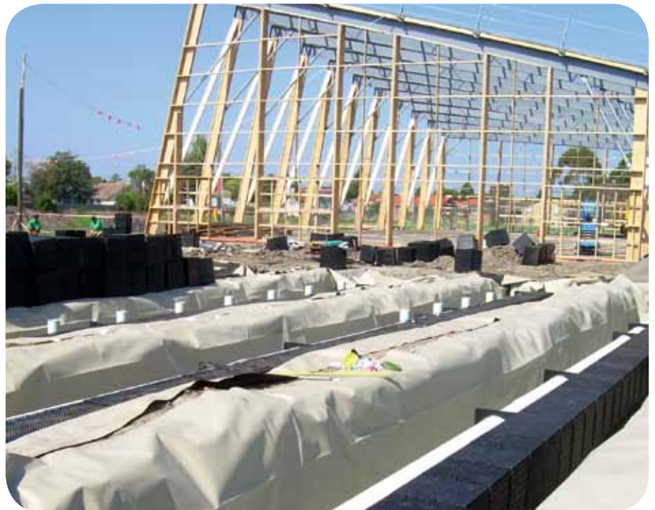
The water-filled foundations were covered during construction.
