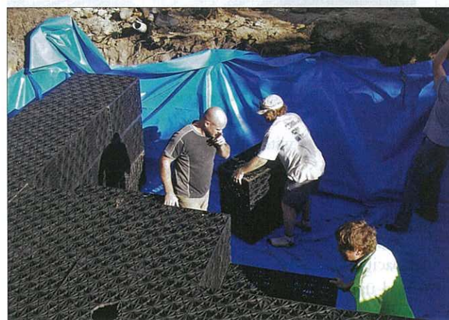
Left: A 30,000 litre underground rainwater tank made from 'milk crates', a polypropylene liner and geotextile fabric was also installed; Right: The new permaculture garden on top of the old pool, now used as a water storage/household cooling system.
